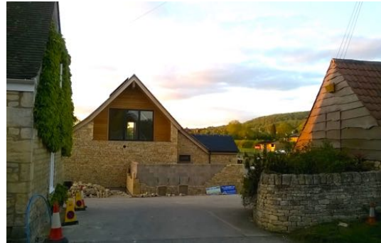
HOME FARM – NEW BUILD
