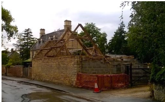
MILL STREET – BARN RENOVATION
