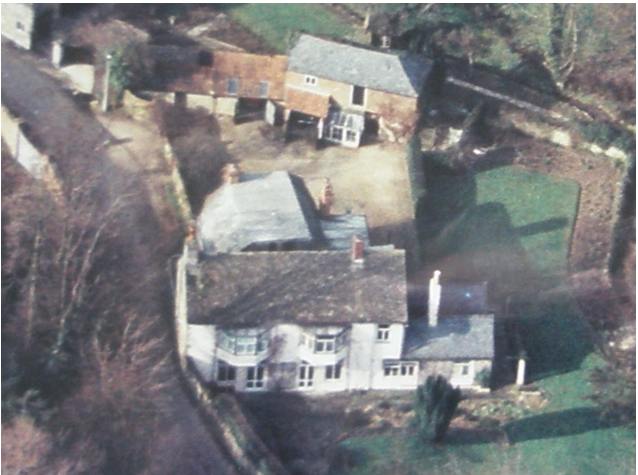
Aerial view (1950s?) of the Lower Mill showing the east front of the house. The single story extension is now two story. It would seem likely that the buttress in line with the chimney was the base of the old chimney and that the north wall of the two story older building was the gable to which the wheel was attached. The millpond reached the fir tree and rockery—the photo conceals the drop of several feet at that point.
